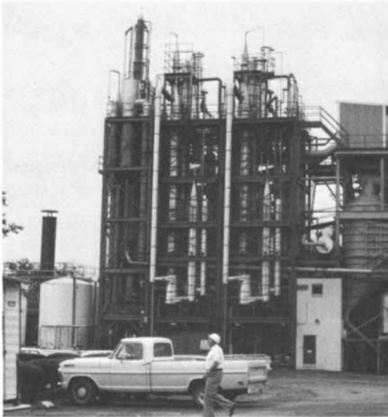
Figure 2. TASTE evaporator (courtesy of George Craddock)
